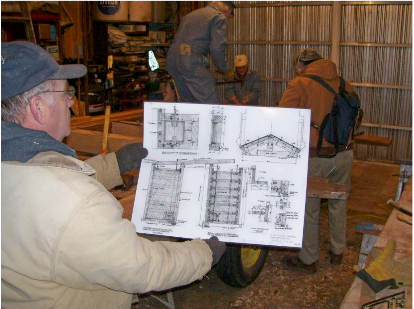
Volunteer Dave Smith reviews plan for the guard lock gate being built in Ed Gruber's barn.
