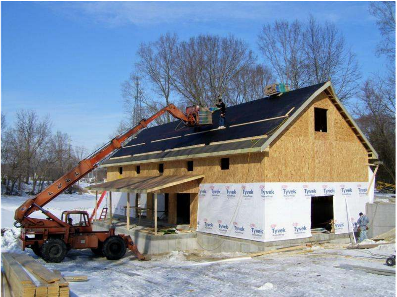
What looks like a porch is actually the "Dock" attached to the warehouse. The three doorways will have full mural paintings that illustrate loading of a canal boat indoors as one might have experienced in 1850.
