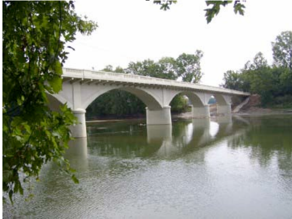
Carrollton Bridge as it looks today
